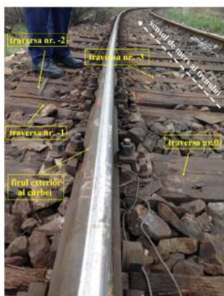
defectele traverselor nr.0 – -3 capetele traverselor dinspre firul exterior al curbei
